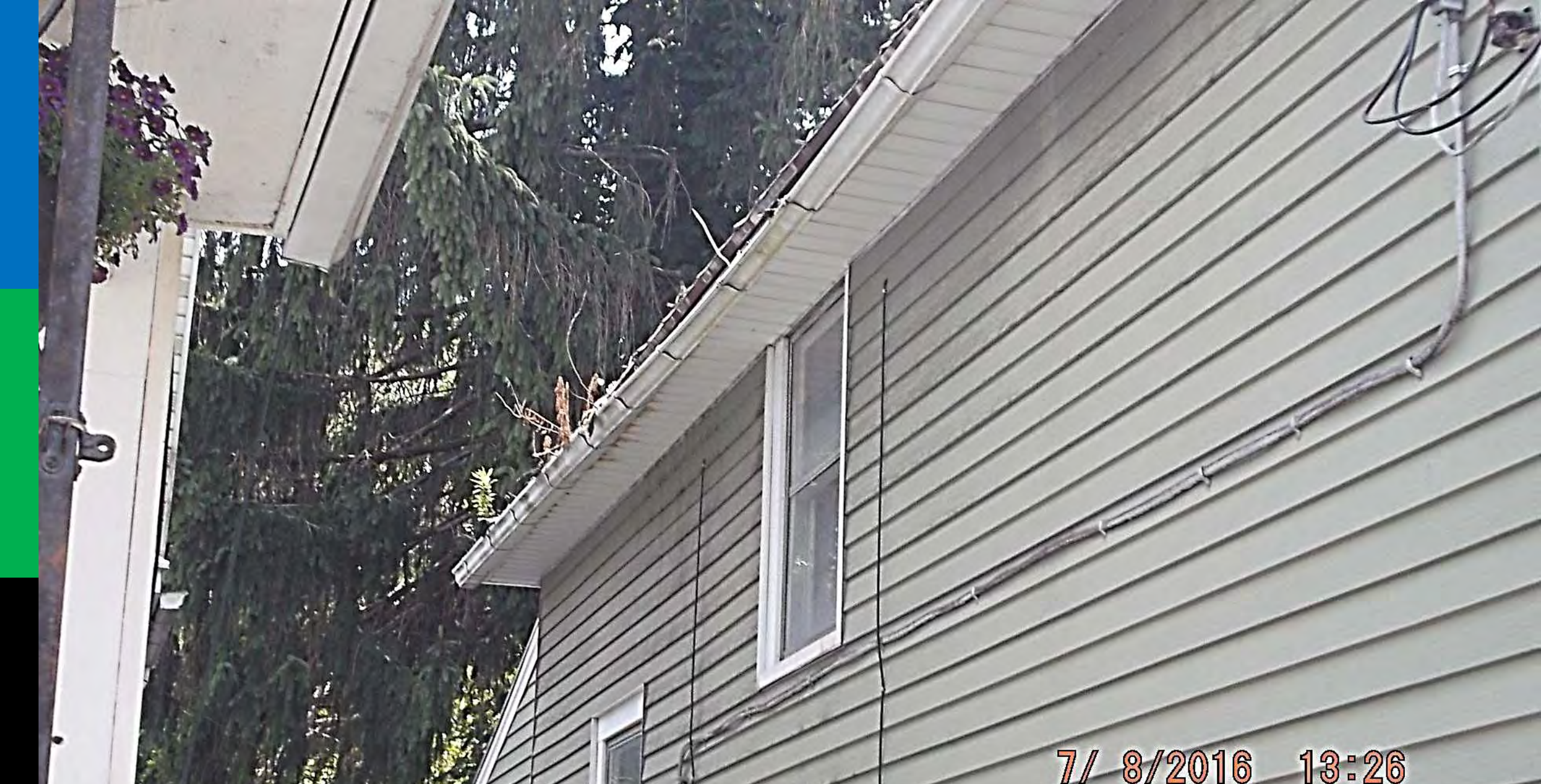
Bank of America failed to clear the gutters so when it rains the water can back up into the roof or damage the walls of the home.
