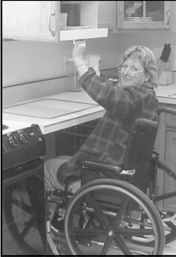
Wheelchair space under counter and stove with controls in front
