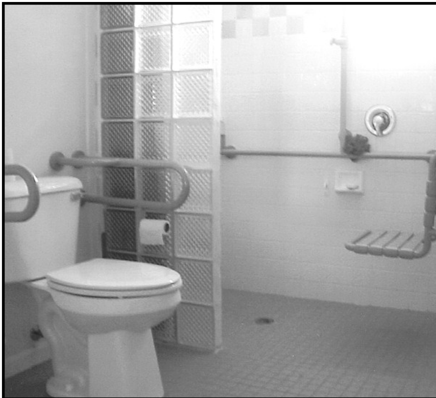
Roll-in shower and toilet with grab bars
